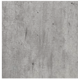
Grey Shuttered Concrete [Wood]
